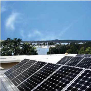
The first stage of the gallery's strategy occurred in 2011 when Lake Macquarie City Council installed 162 photovoltaic cells and a voltage reduction unit at the gallery, resulting in 20 per cent less energy used annually. This second stage will be the installation of specialist LED lighting and digital dimming system. The new lighting system will generate an estimated further 10 per cent savings in overall energy use annually.
